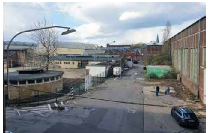
View onto the Osthof courtyard, 2023
